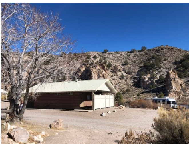
Showers / Bathroom- Sam Stowe Campground
